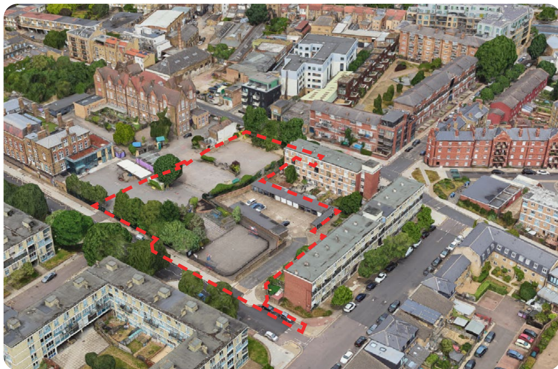
Aerial View of Site from South East, prior to Demolition Works
