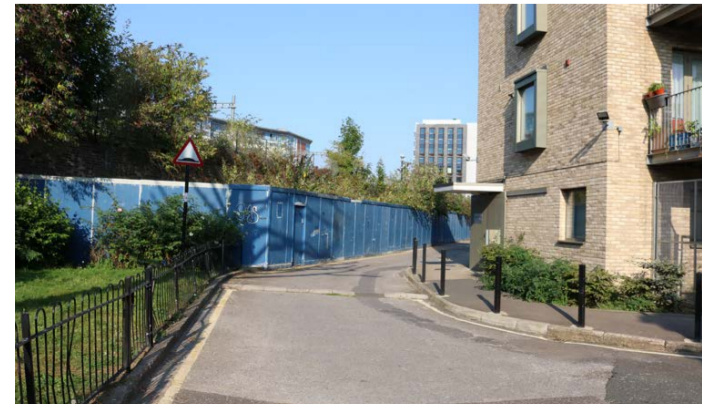
07. View along Bradwell Street
