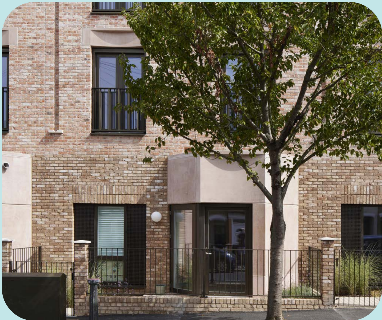
Brickwork facade Gort Scott, Walthamstow
